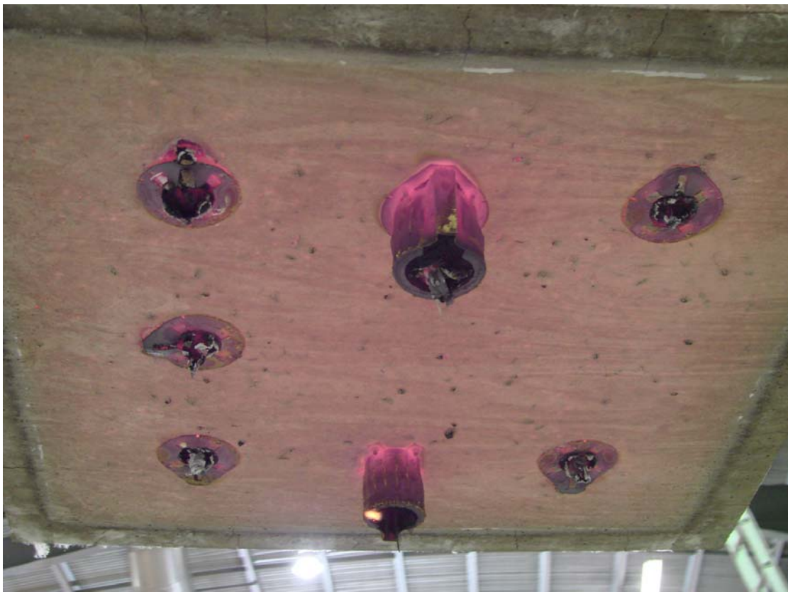
Photograph 14 – Exposed face after the conclusion of testing
