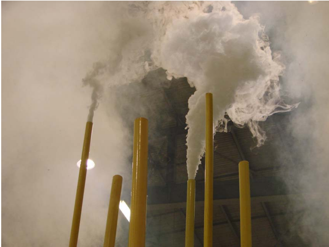
Photograph 3 – End of pipes after 8 minutes of testing
