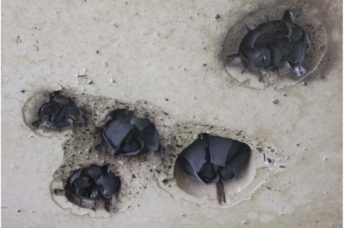
PHOTOGRAPH 7 – EXPOSED FACE OF SPECIMENS AT CONCLUSION OF TESTING
