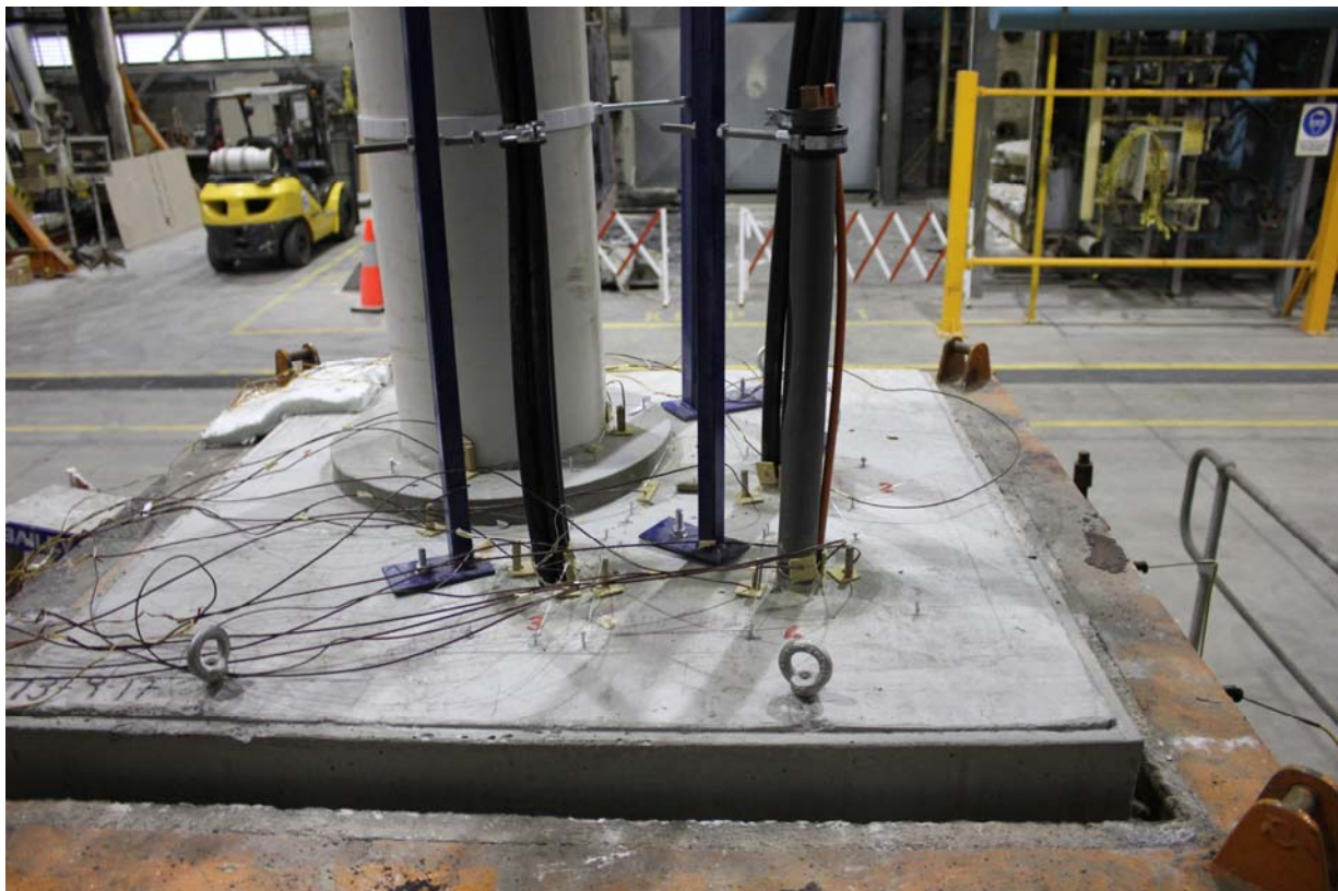
PHOTOGRAPH 2 – UNEXPOSED FACE OF PENETRATIONS PRIOR TO TESTING
