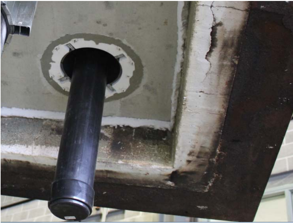
PHOTOGRAPH 1 – EXPOSED FACE OF SPECIMEN 2 PRIOR TO TESTING
