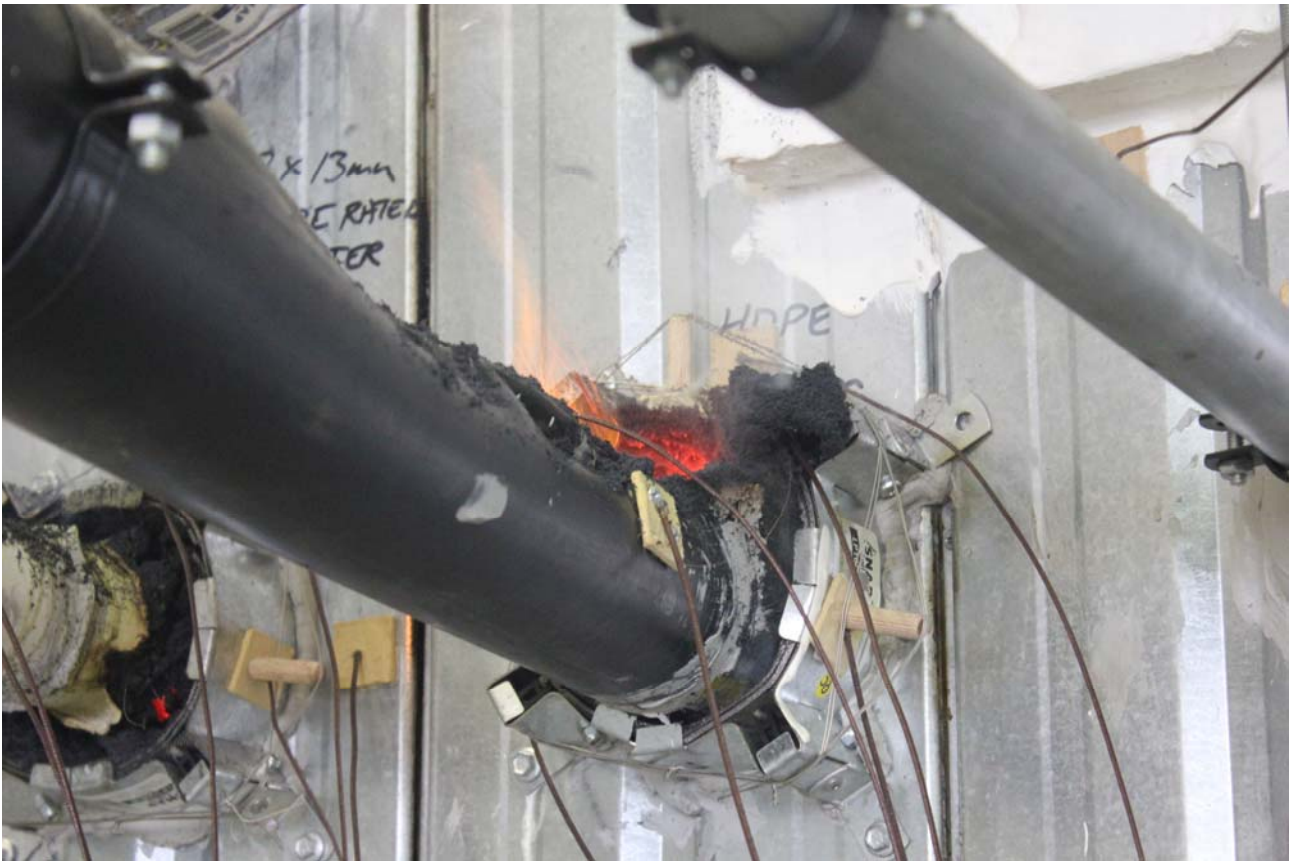
PHOTOGRAPH 9 – SPECIMEN 12 AT 80 MINUTES INTO THE TEST
