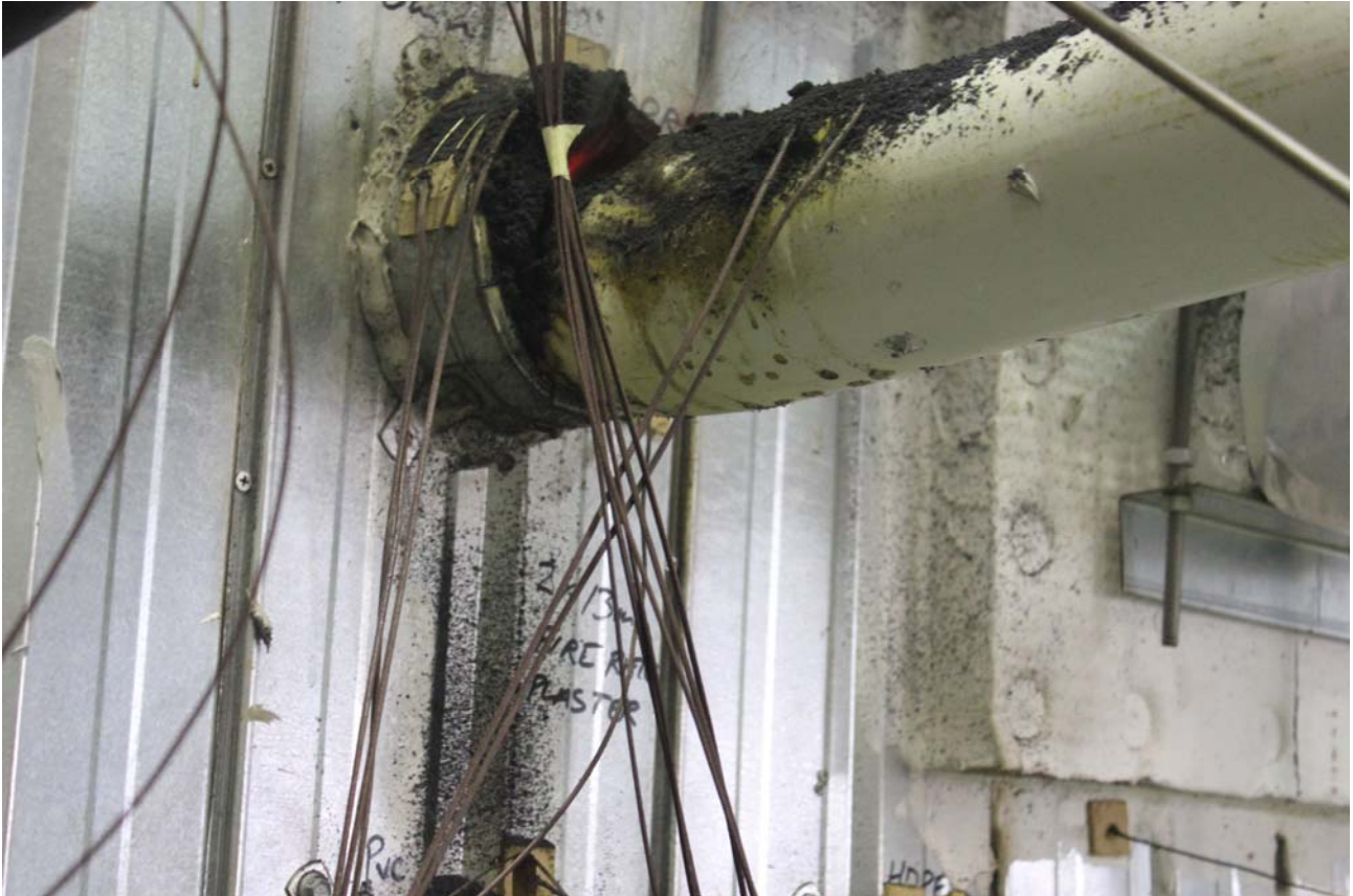
PHOTOGRAPH 12 – SPECIMEN 10 AT 113 MINUTES INTO THE TEST
