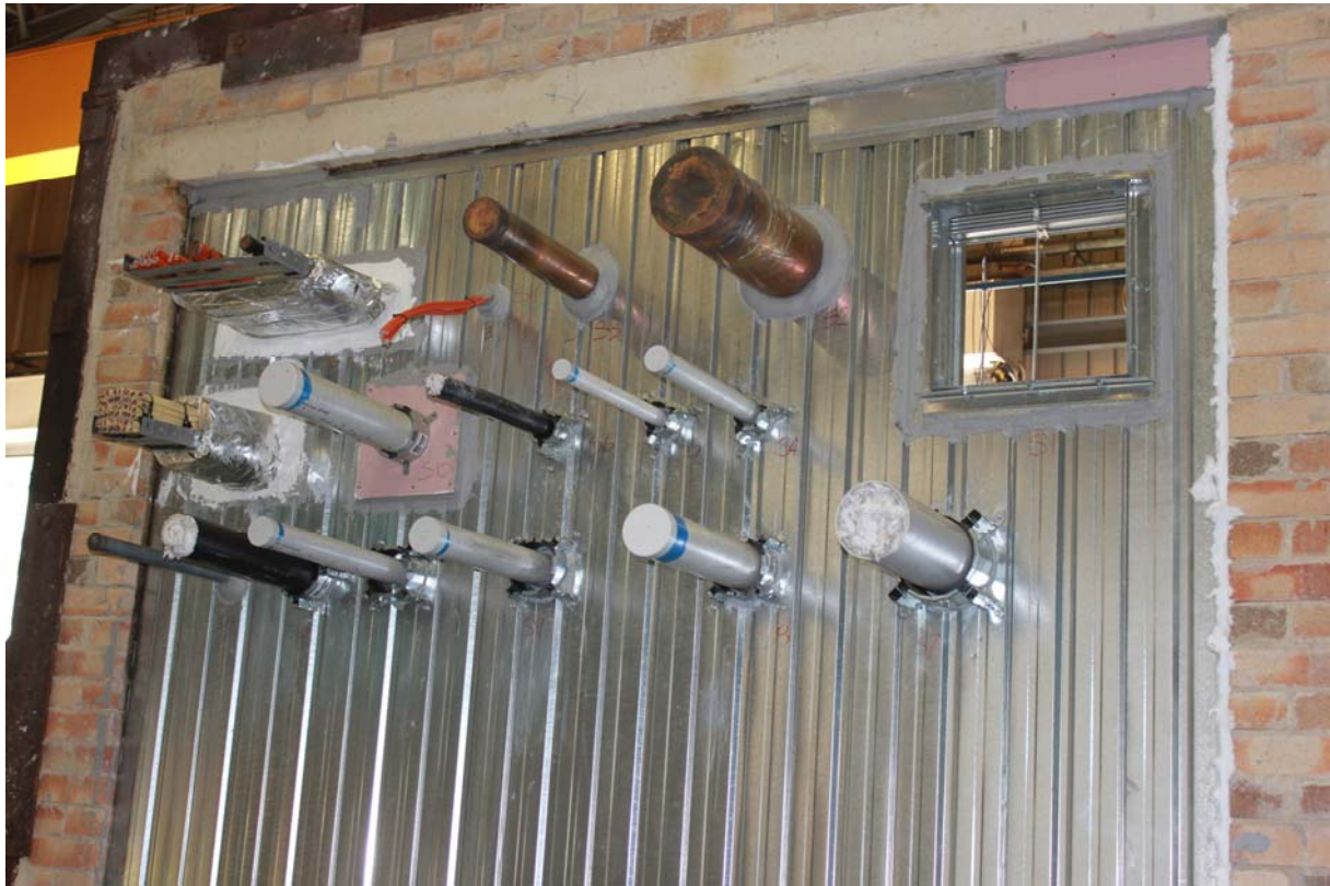
PHOTOGRAPH 1 – EXPOSED FACE OF THE SPECIMEN PRIOR TO TEST
